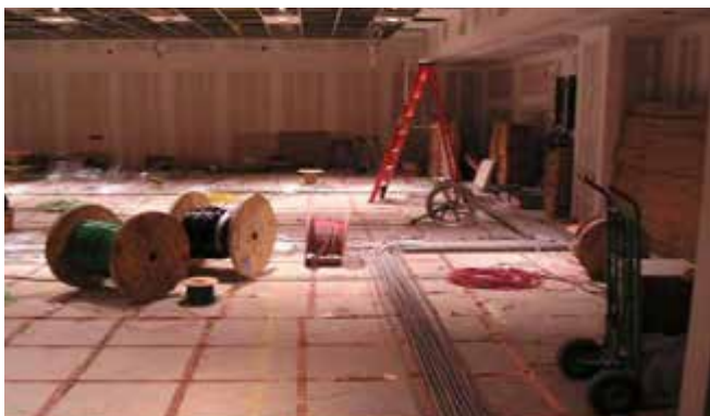
Command and Control Facilities
