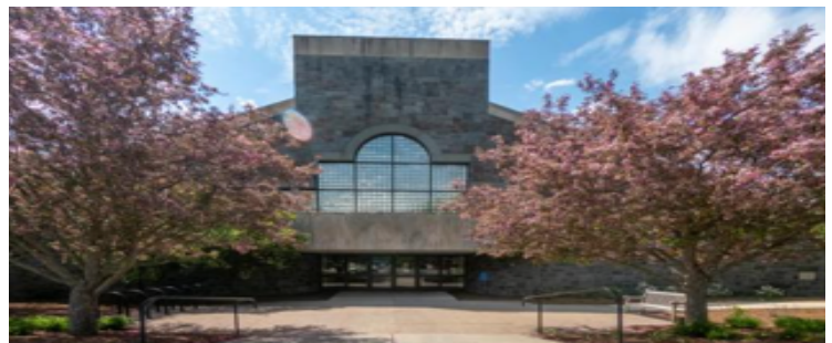
Sanford Fieldhouse - Security Alterations
